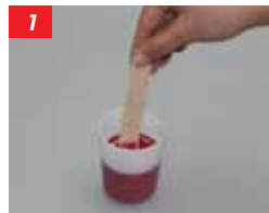
1 Make up the paint formulation from the Mastermix system. Check the colour and stir the mixed paint
